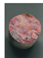
Concrete Core Moisture Advanced ASR
